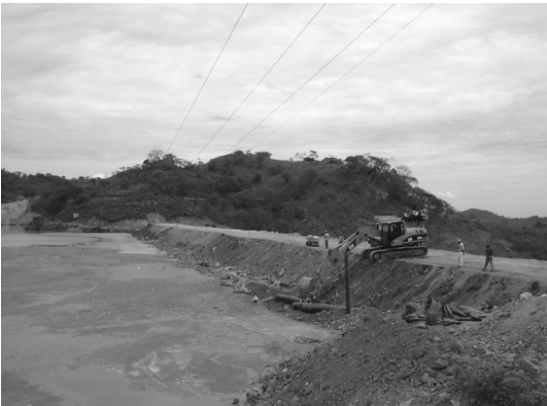
Figure 14. View of the completed Phase IV crest raise, looking downstream.
