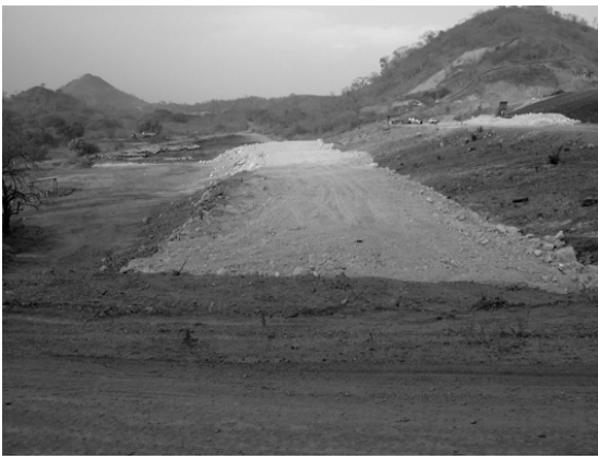
Figure 9. View of the Phase IV keyway/toe buttress.
