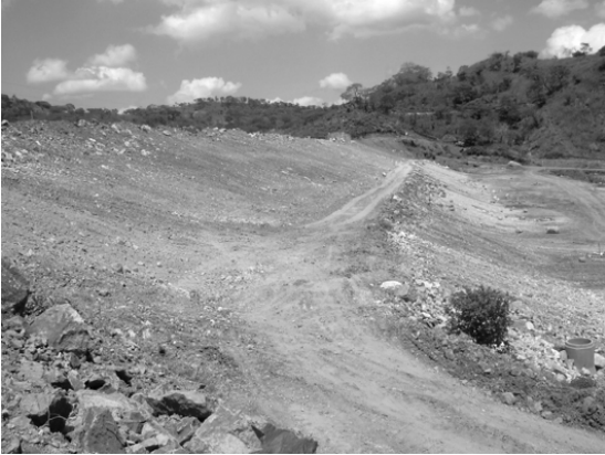
Figure 13. View of the completed Phase IV downstream rockfill shell.
